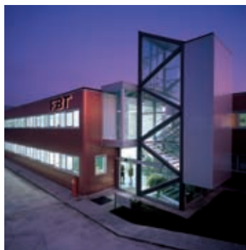
The entrance to FBT offices
